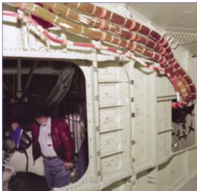
Figure 4.2-3. Typical wiring bundle inside Orbiter wing.
